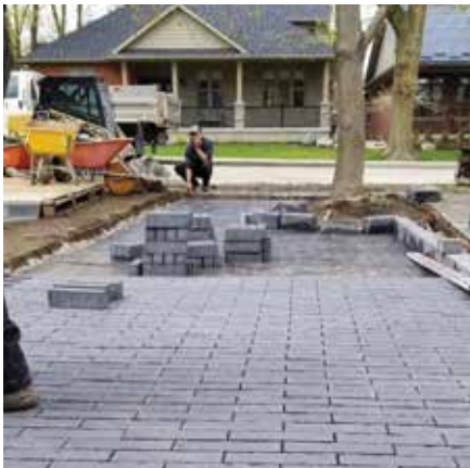
"You stage pavers throughout the job without damaging your prep work. Big time savings!"
